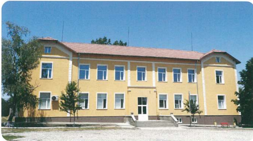
Introduction of energy efficiency measures in the building of „Vasil Levski“ Primary School, Enitsa village, Knezha municipality
